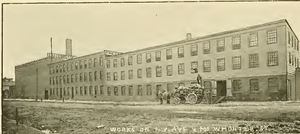
WORKS ON N. Y. AVE. & McWHORTER ST.
